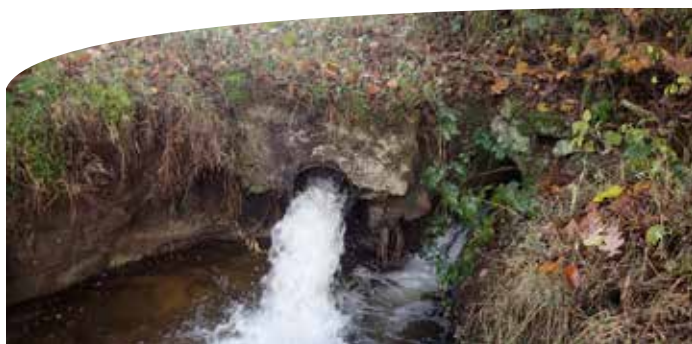
Fig.6 buse infranchissable
